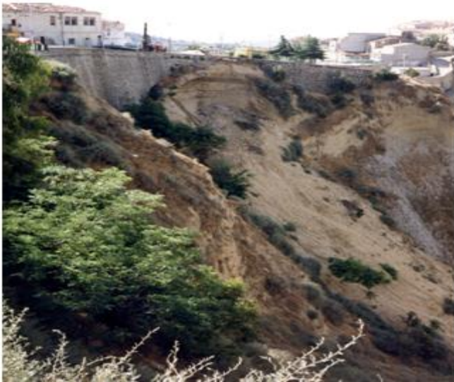
Figure 6: Example of mudflow landslide in Aliano built-up area in Basilicata region activated by the earthquake on 23 November 1980
