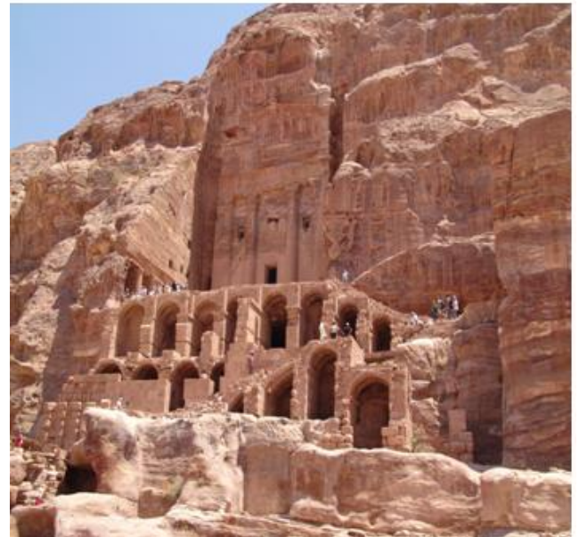
Figure 8: Erosion and rock falls at the Tomb of the Urn Complex in Petra
