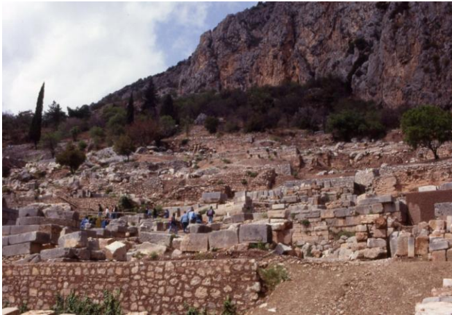
Figure 12: Overview of Delphi's archaeological area with wide outcrops of debris and collapses occurred in fractured limestones
