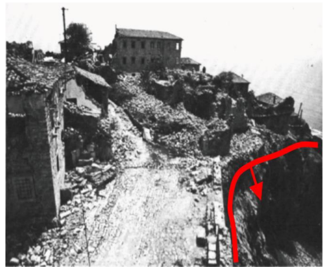
Figure 14: Historical image representing the half-destroyed village upstream of Cattaro because of an earthquake occurred on May 29, 1979. On the right, rockfalls triggered by the earthquake are also showed
