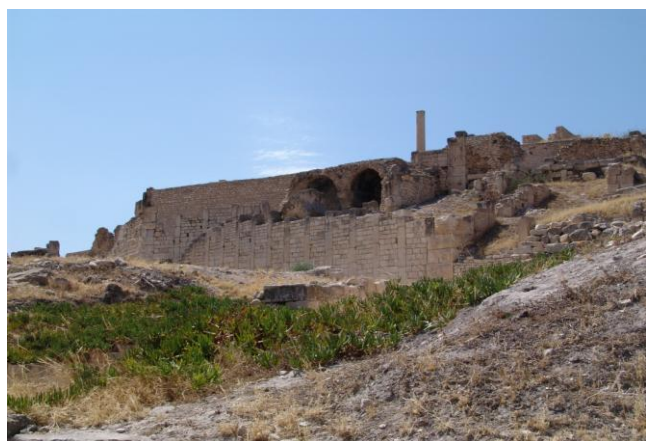
Figure 10: Appearance of the unstable area with ancient retaining walls (Dougga). In the foreground the outcrop of plastic clays is seen
